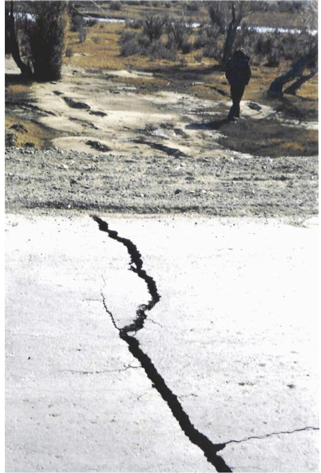
**Figure 23.** Gryphons on the extension of a seismic-vibration fissure in the Kosh-Agach-Beltir road.
